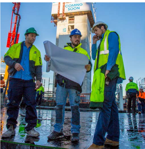
Apartment construction in Chatswood
