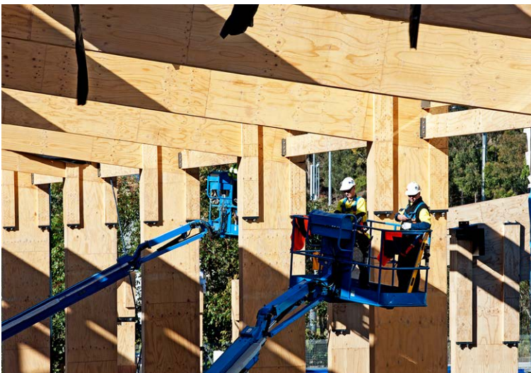
Netball facility under construction, Parramatta
