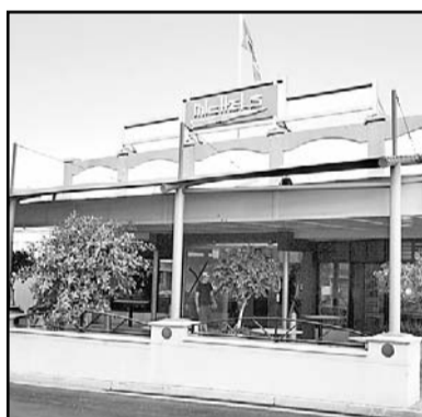
Michels Cafe and Bar refurbishment
